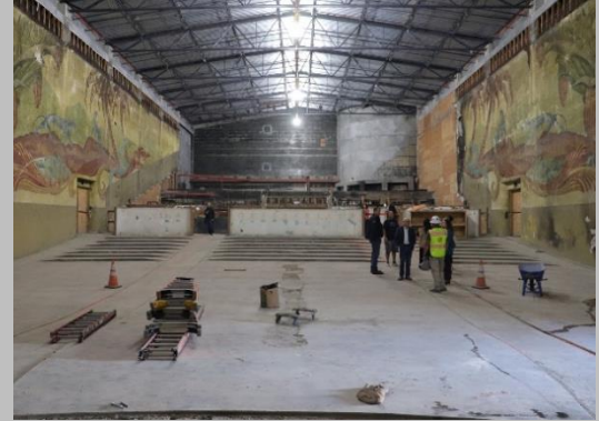
RENOVATION IN PROGRESS
