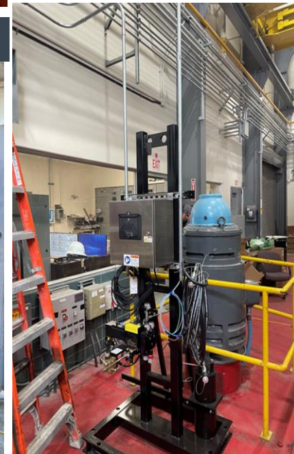
REXA Electraulic Actuator Installation
